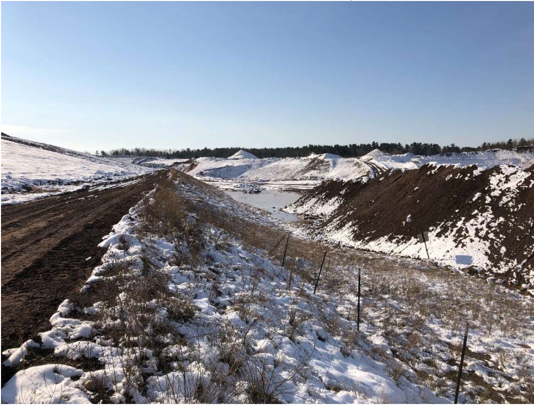
Location 4 – Looking South, Phase 3 Western Berm
