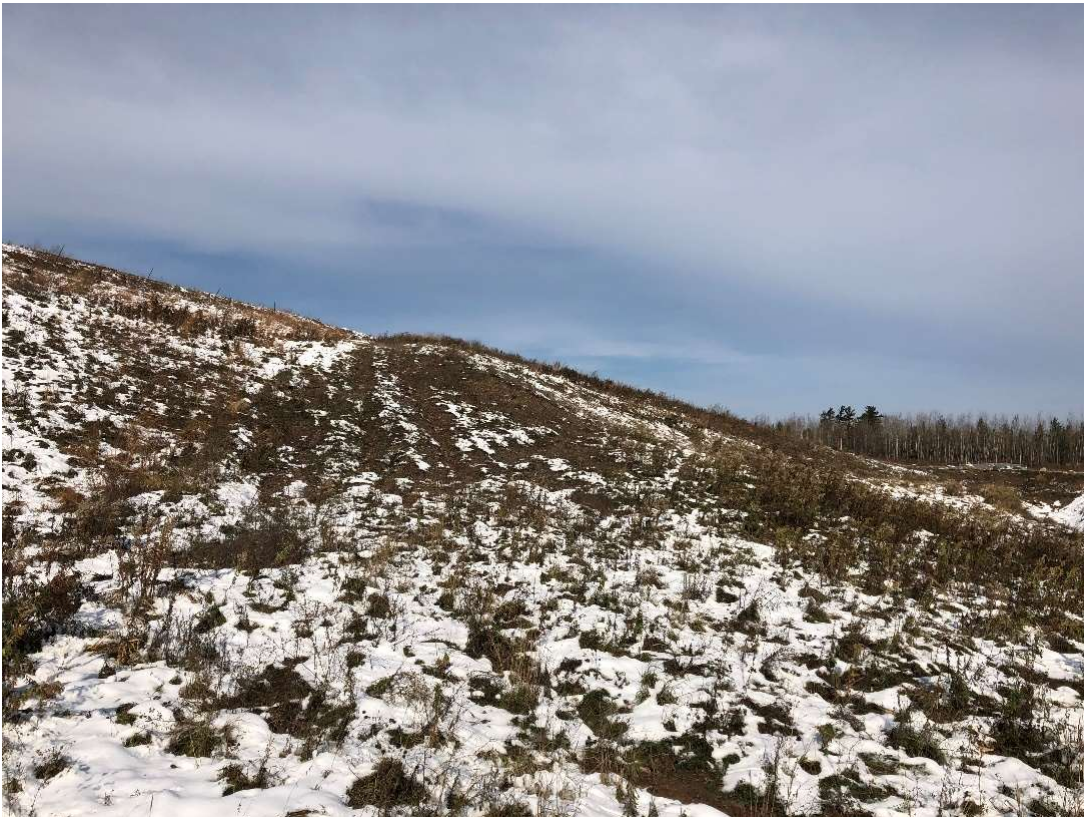
Location 11 – Looking North, Phase 1 Northern Access Road
