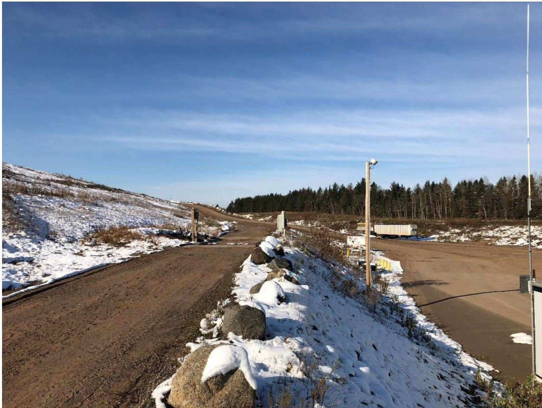
Location 1 – Looking West, Phase 1 Northern Berm
