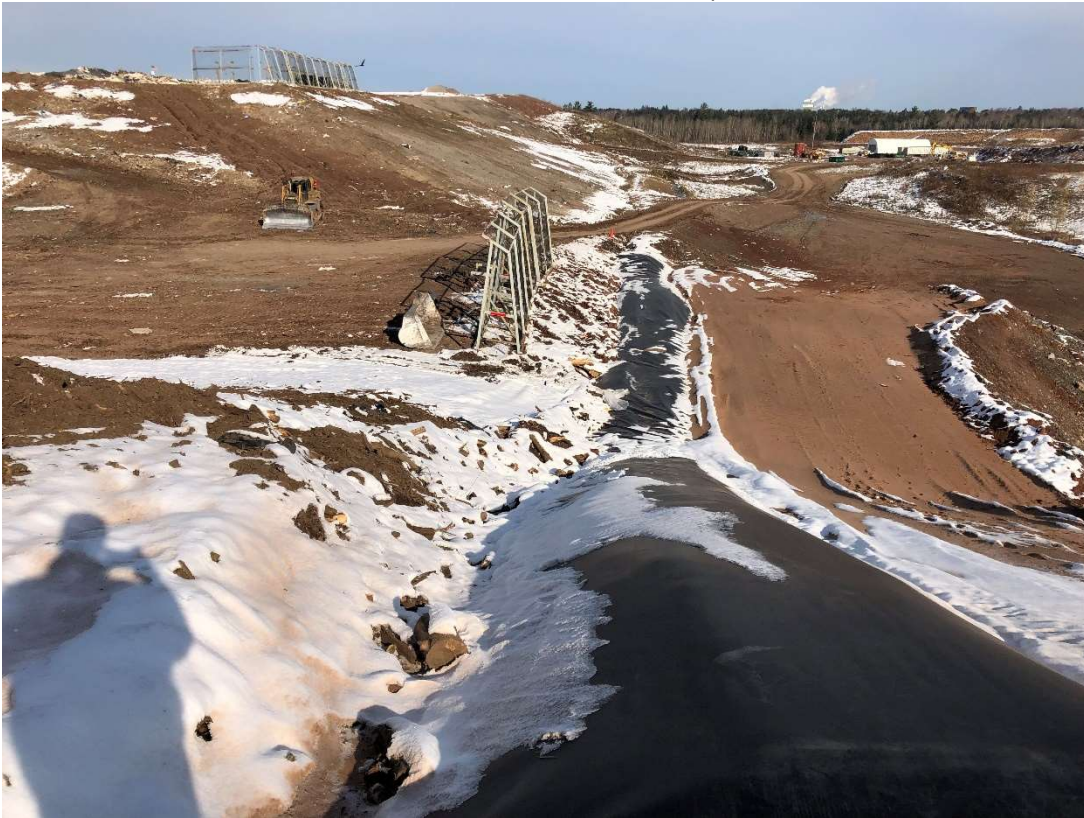
Location 8 – Looking North, Cell 6 Eastern Anchor Trench
