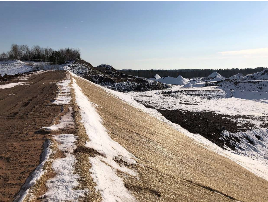
Location 7 – Looking East, Cell 6 Southern Berm
