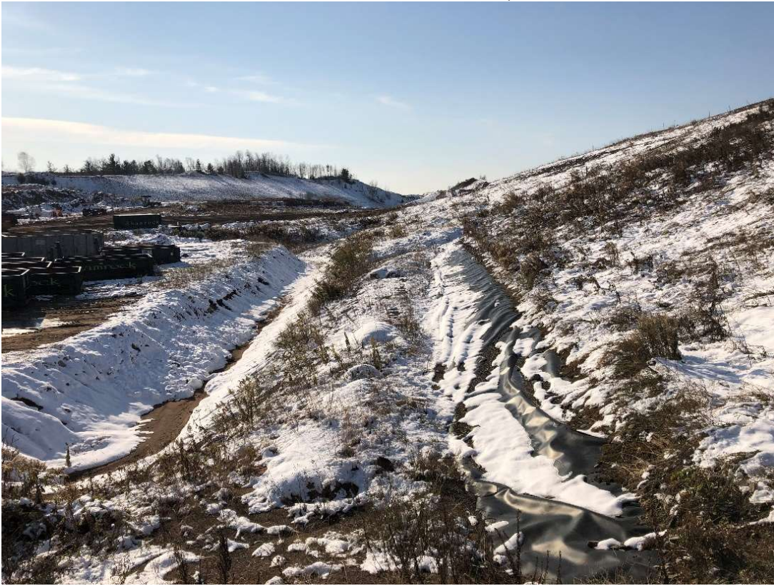
Location 1 – Looking South, Phase 1 Eastern Berm
