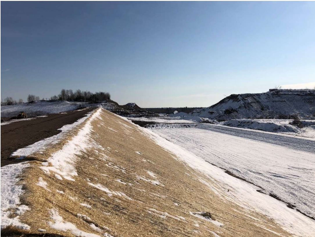
Location 6 – Looking East, Phase 5/6 Southern Berm
