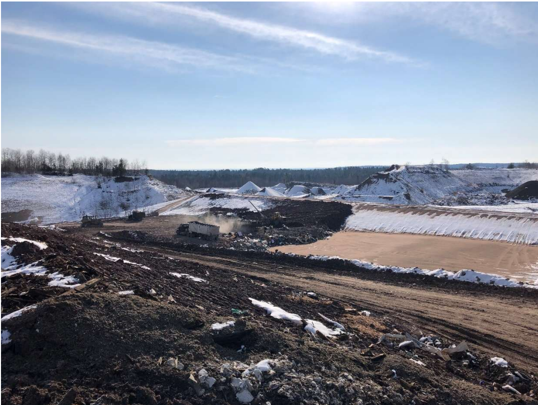
Location 13 – Looking Southeast, From Phase 3 Upper Lifts At Phase 5/6
