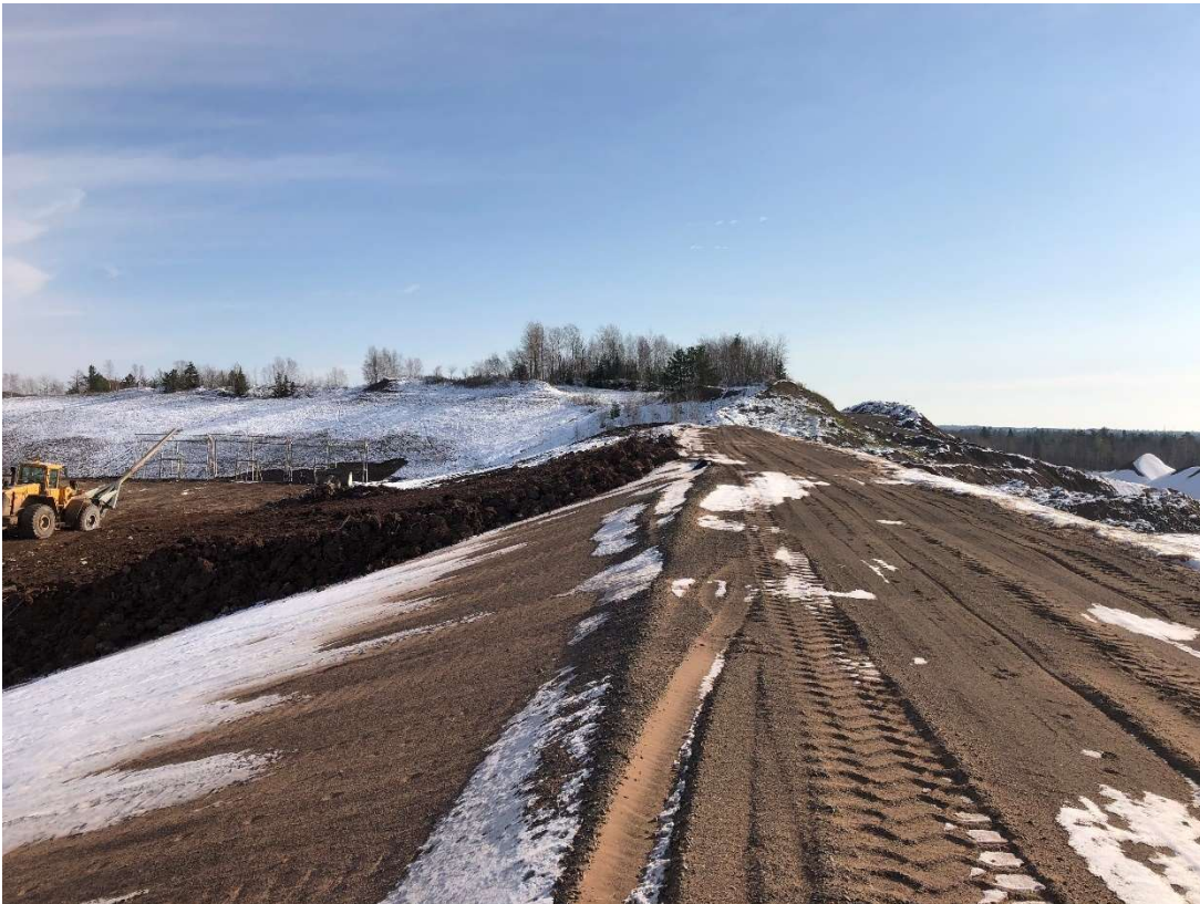
Location 7 – Looking East, Cell 6 Southern Anchor Trench
