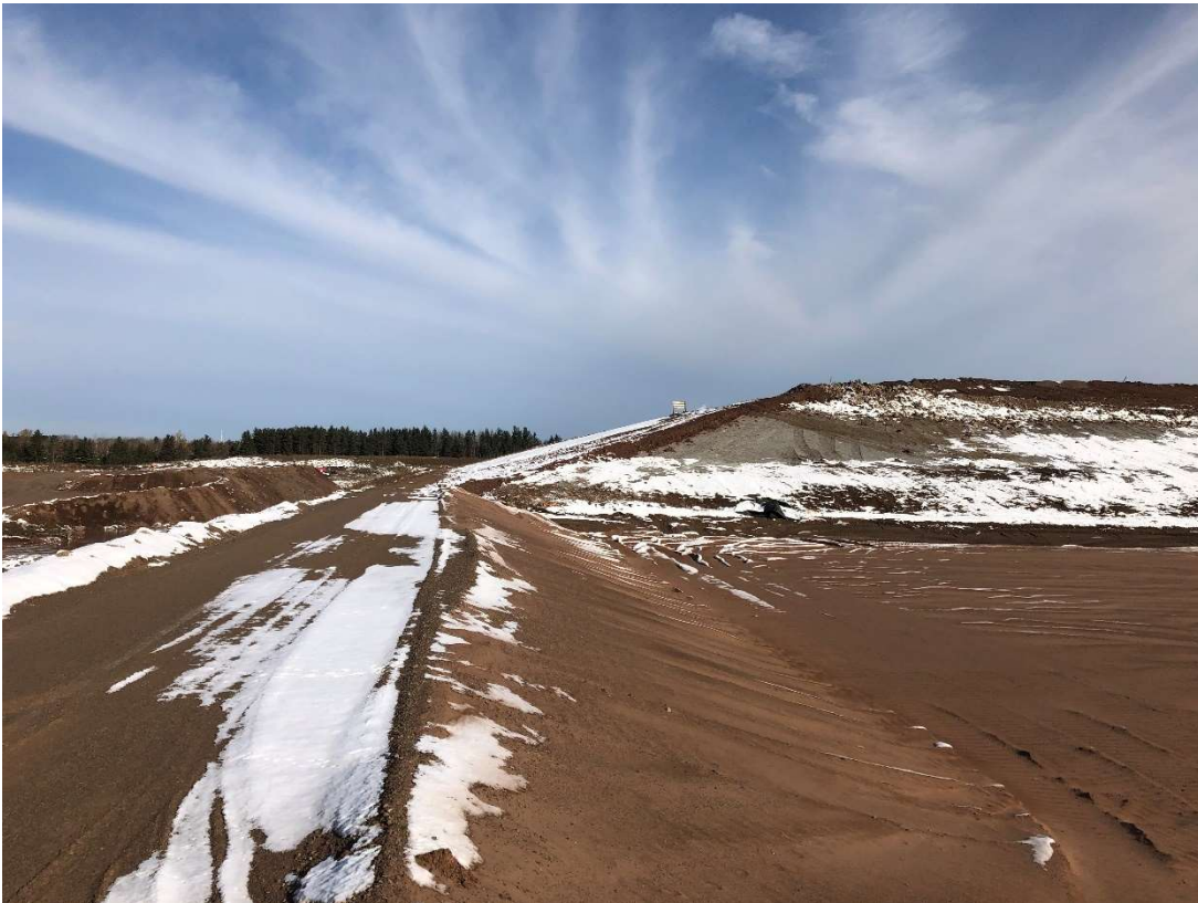
Location 6 – Looking North, Phase 6 Interior (Future Waste Slope)
