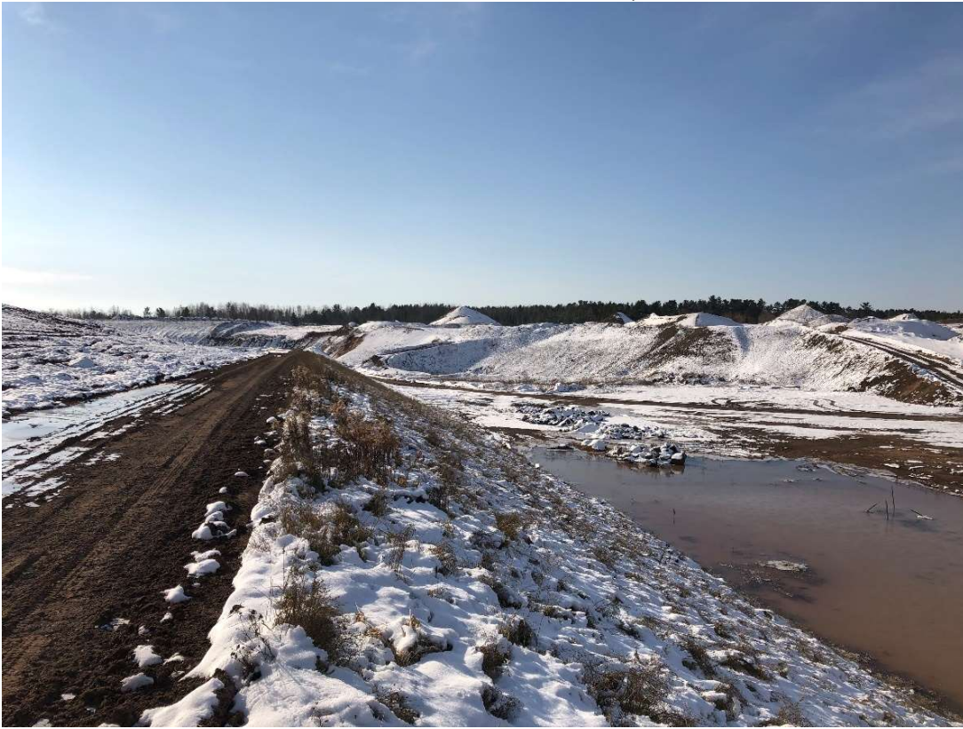
Location 5 – Looking South, Phase 6 Western LF Berm
