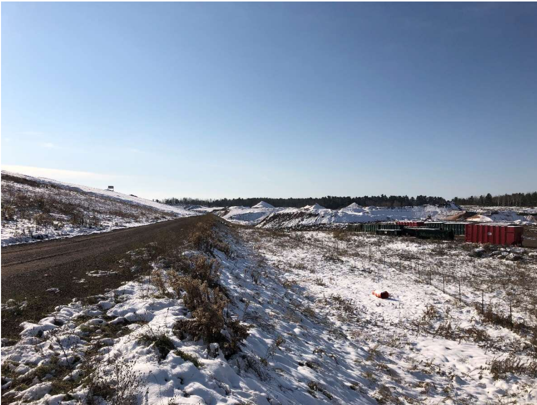
Location 3 – Looking South, Phase 2 Western Berm
