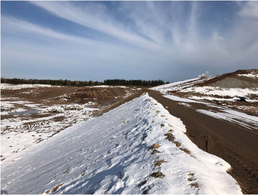
Location 6 – Looking North, Phase 6 Western LF Berm
