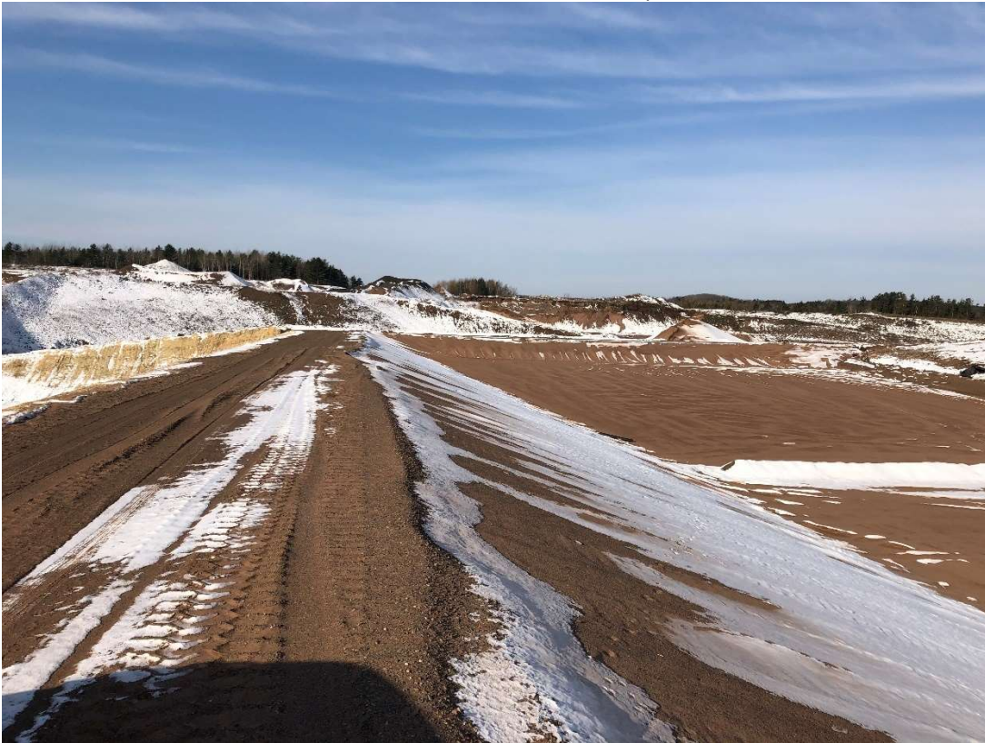
Location 7 – Looking West, Cell 5 Southern Anchor Trench
