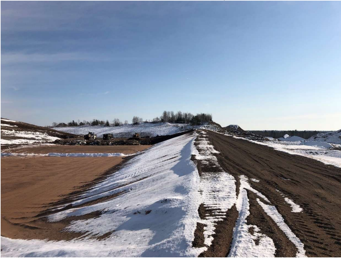
Location 6 – Looking East, Phase 5/6 Southern Anchor Trench
