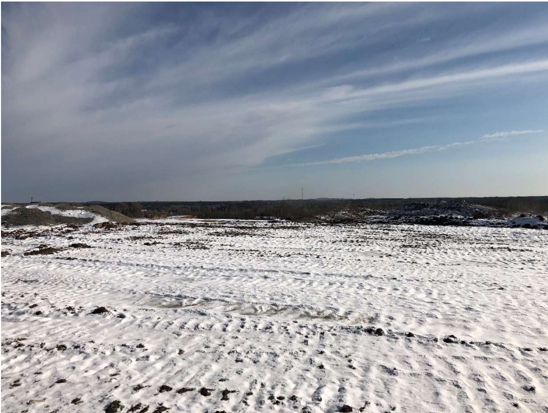
Location 12 – Looking East, Phase 2/1 Upper Lifts
