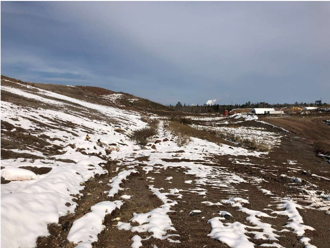
Location 9 – Looking North, Cell 6 Eastern Anchor Trench
