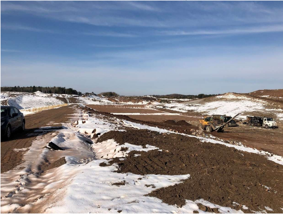
Location 8 – Looking West, Cell 6 Southern Anchor Trench
