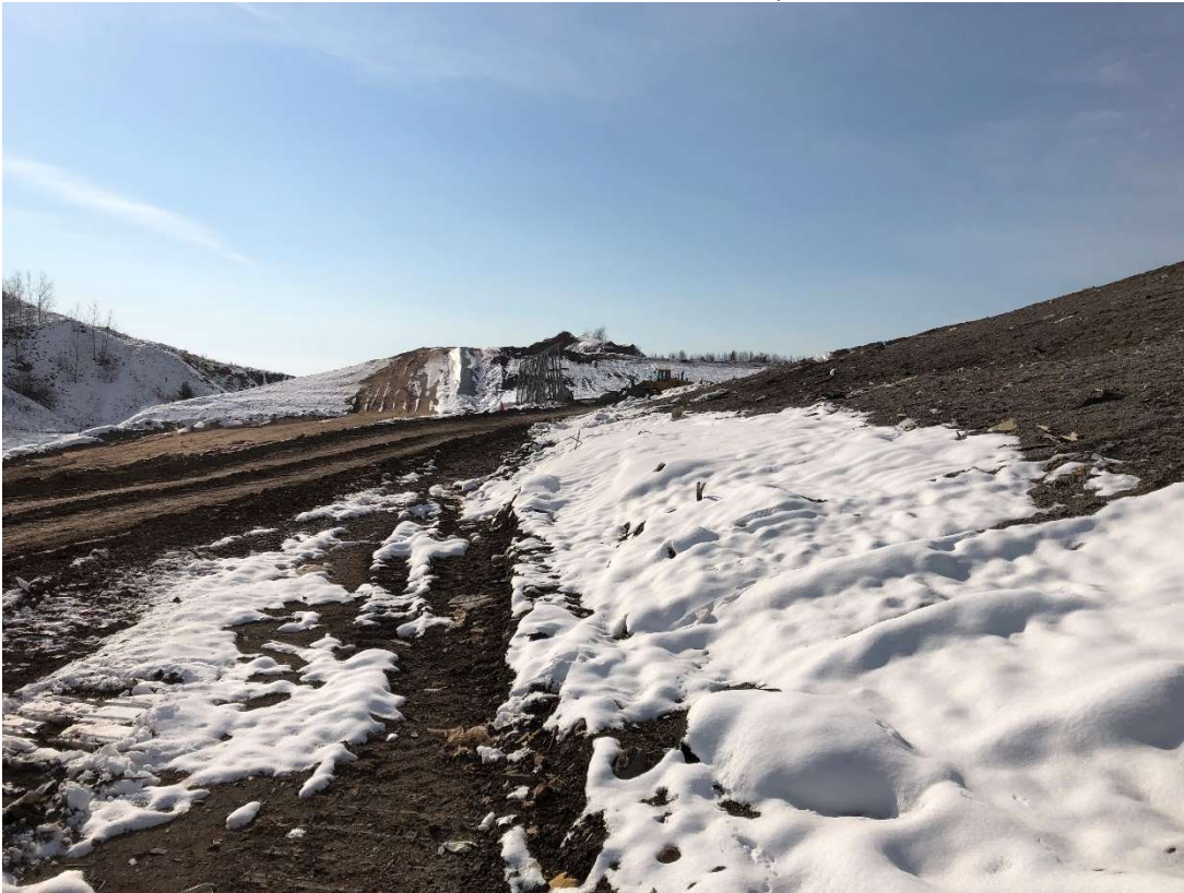
Location 9 – Looking South, Cell 6 Eastern Anchor Trench
