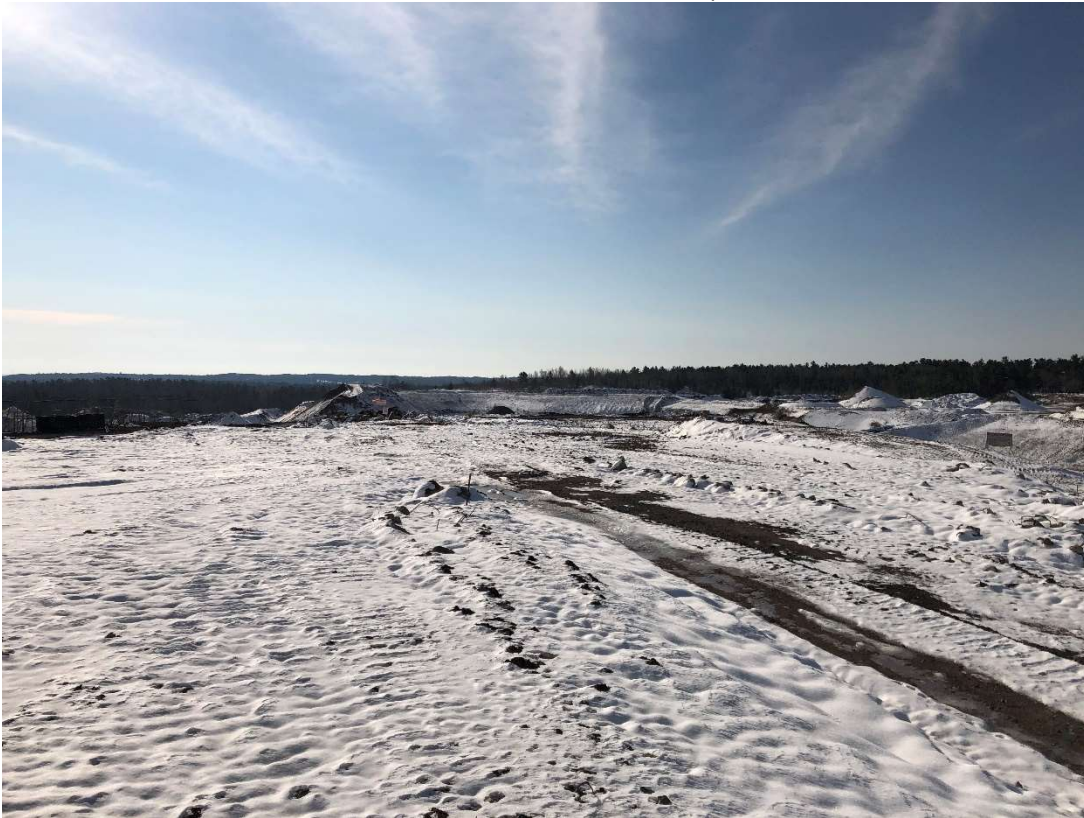
Location 12 – Looking South, Phase 2/3 Upper Lifts
