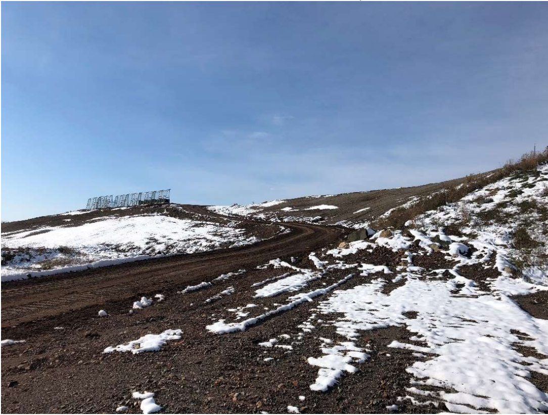
Location 11 – Looking Southwest, Phase 1 Southern Access Road
