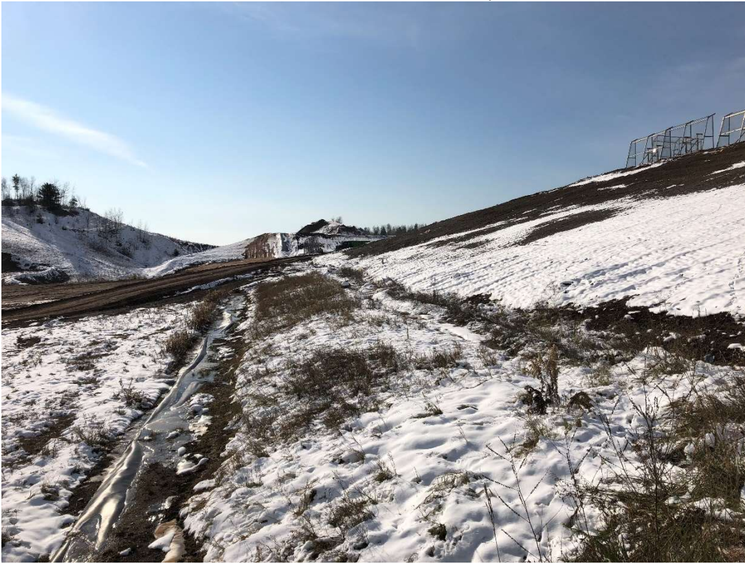
Location 10 – Looking South, Phase 4 Eastern Berm and Waste Slope
