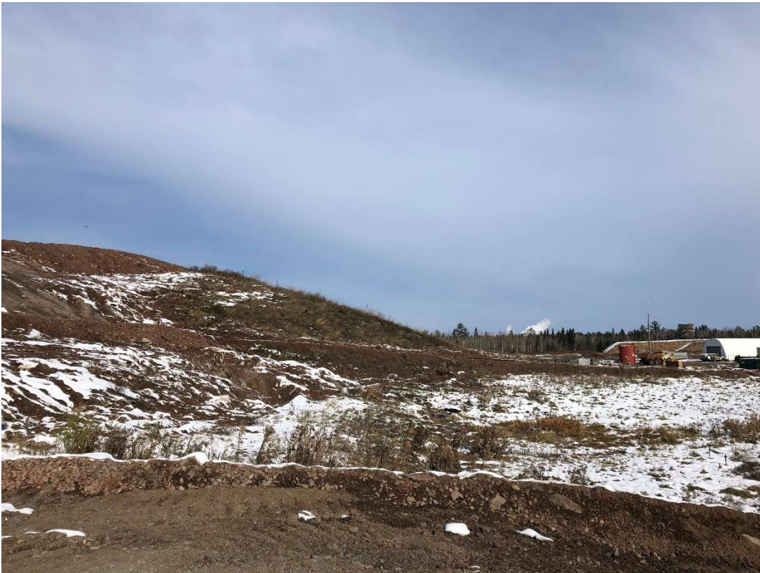
Location 10 – Looking North, Phase 4 Eastern Berm & Phase 1 Southeast Corner
