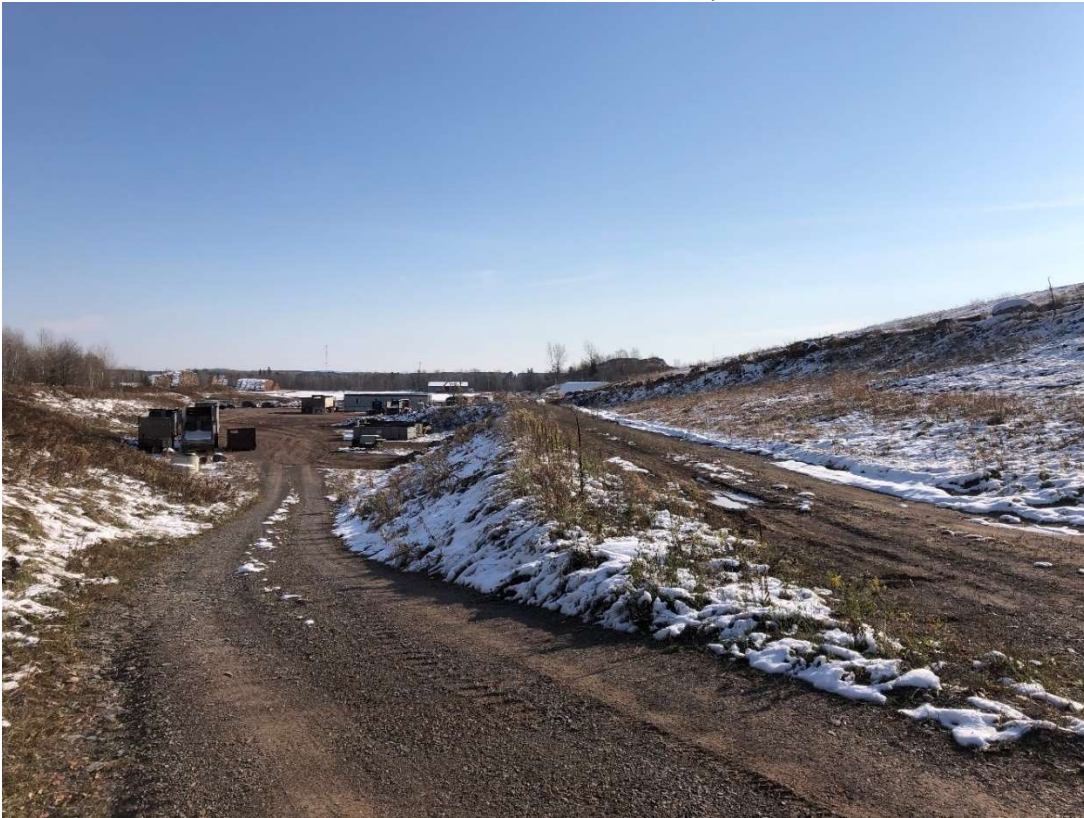
Location 3 – Looking East, Phase 2 Road & Berm
